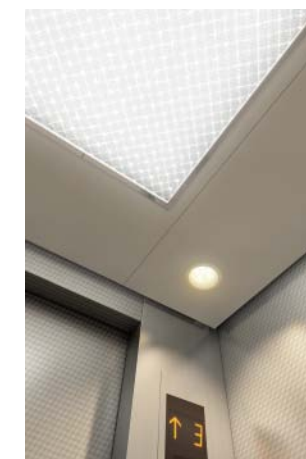
Ceiling: Painted steel sheet (Y033) with an acrylic lighting cover Lighting: Central lighting and downlights (LEDs)
